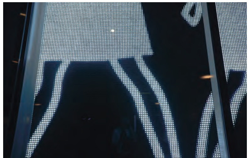
Fig. 6: Close-up view of the low resolution pixel pitch. Photo: J. Hartmann.
